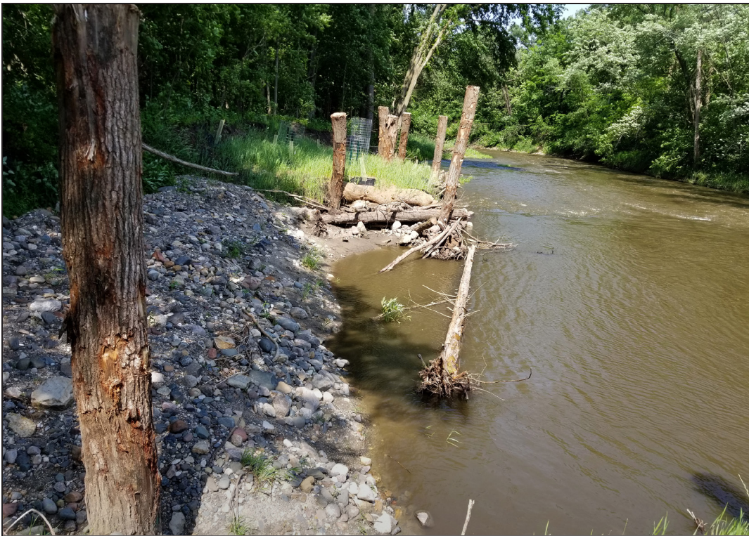
Between the root installations are a series of bays. The project is seen from farther downstream.
