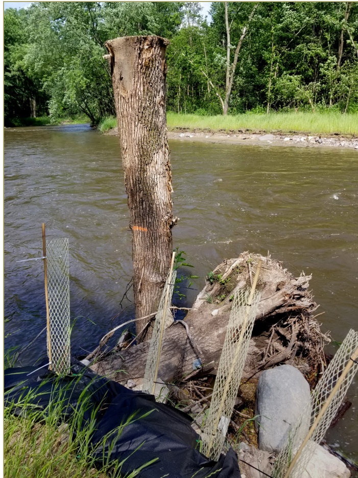
Bolts hold tree trunks and roots in place along a bend in Sand Creek, where fast-moving water has caused erosion.
